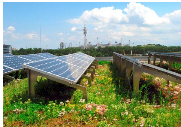
Slim energiedak in Rotterdam.
